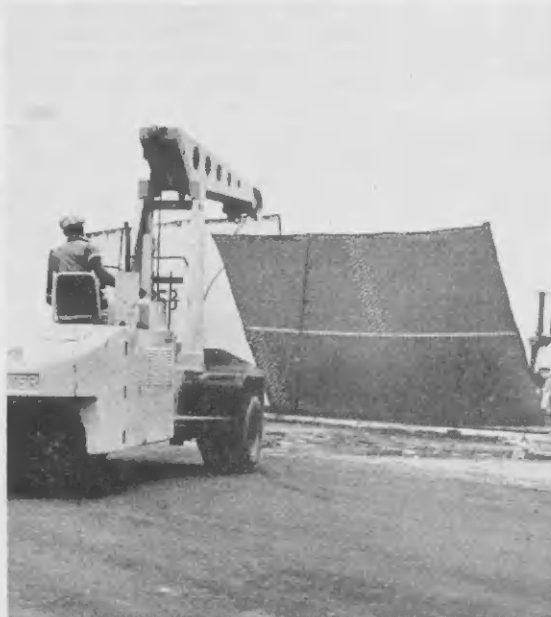
LIKE A dentist pulling teeth, this specialized vehicle jerks out storage tank sections with speed and ease. The steel sections are slated for the scrap pile.
